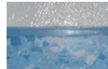
THERMOWELDED DECOCHOC Panel / panel or panel / floor hot-welding
